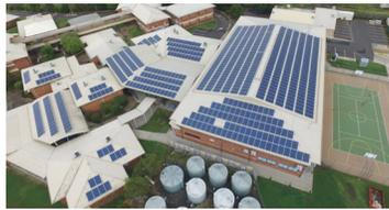
This Bundaberg, Queensland, private school installed a 194kW rooftop solar system with battery storage and upgraded its fluorescent lights to LEDs. Grid energy consumption fell more than 80 per cent and the Large-scale Generation Certificate revenue offsets the school's remaining power bill.
