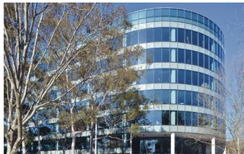
This 25-year old office building in Sydney installed new chillers, variable speed drive pumps, 100kW solar PV, building management system, power factor correction unit and replaced its single glazed façade. The deep retrofit resulted in a PCA A Grade, an increase from a 2.5 Star to 5.0 Star NABERS Energy Base Building Rating and a 35 per cent reduction in carbon emissions.
