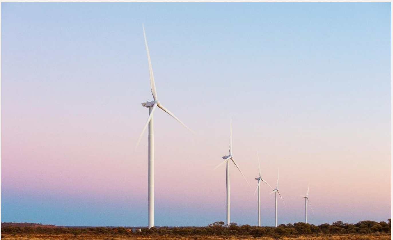
Figure 21: Wind turbines at the Agnew Renewable Energy Microgrid (image courtesy of EDL)
