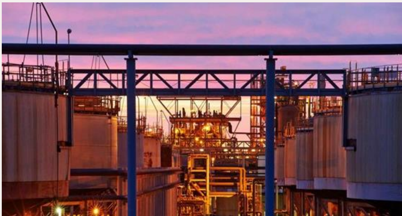
Figure 55: Alcoa's Wagerup Refinery (image courtesy of Alcoa)
