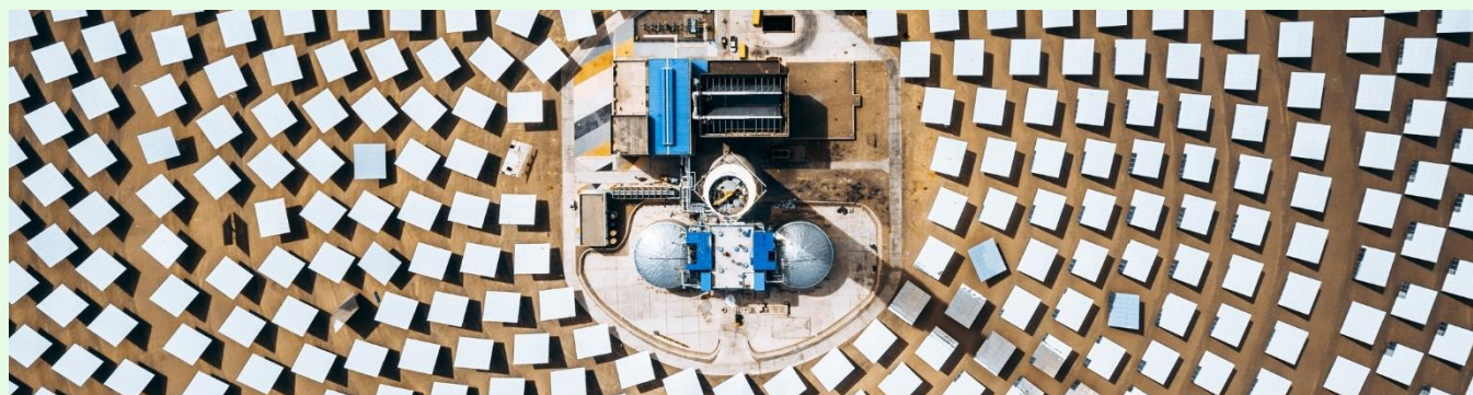
Figure 12: Concentrated solar thermal example being piloted by Rio Tinto on a mine site in California
