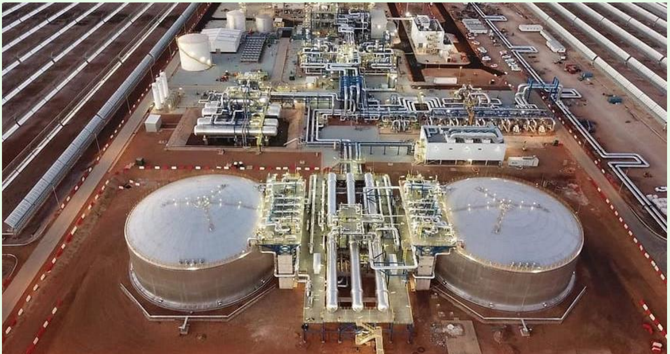
Figure 19: Kathu Solar Park, South Africa, with molten salt storage system (image courtesy of Tractebel, Engie)
