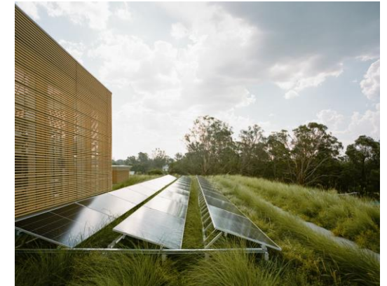
Figure 4. Landscape design of the bio-solar PV roof of First Building – Bradfield City Centre.
